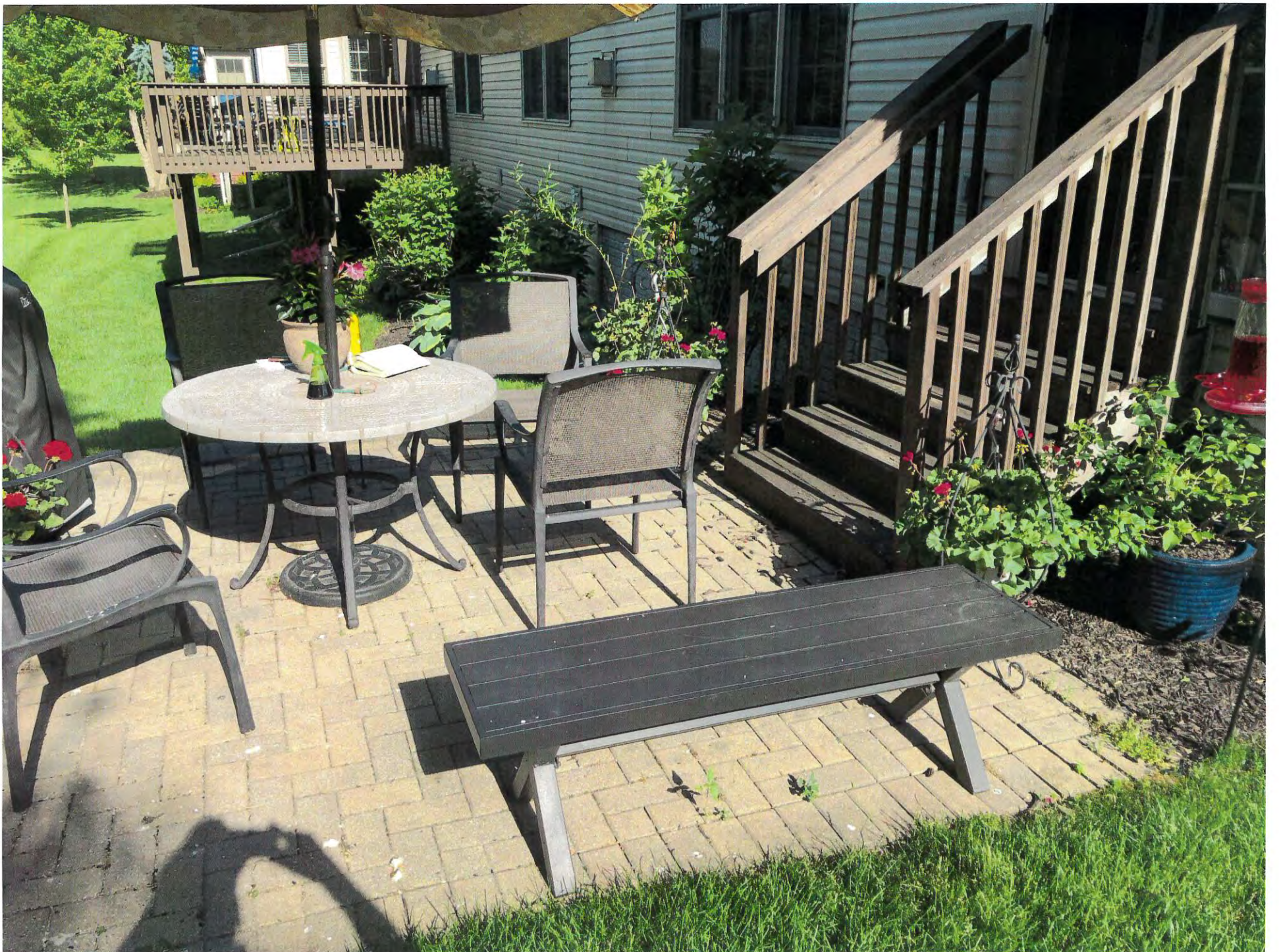
EXISTING PATIO & STAIRS 16' DEEP 12' WIDE
